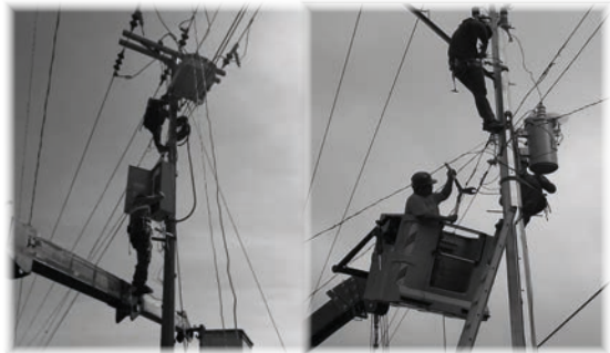
Installation of Distribution Transformers and Reclosers
