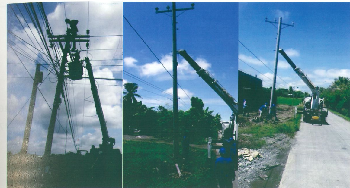
UPGRADING OF DISTRIBUTION LINES
